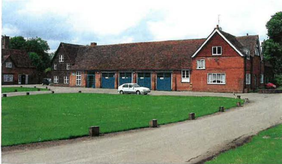
Fig. 38 Barns - view from south.
