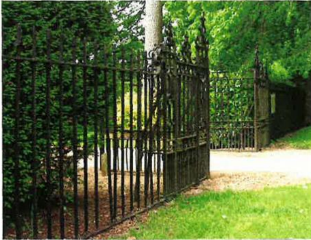
Fig. 9 Main entrance gates and fence screen.
