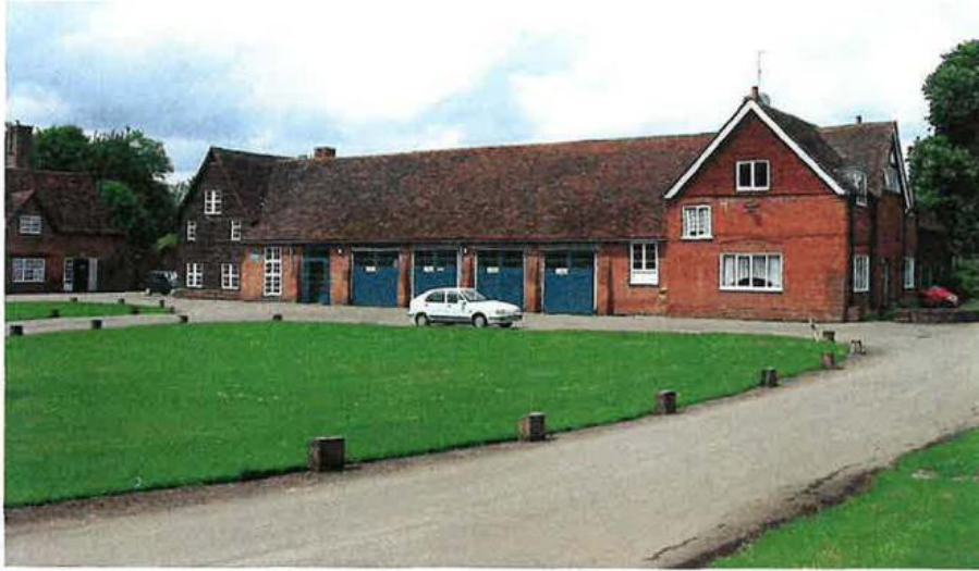
Fig. 38 Barns - view from south.
