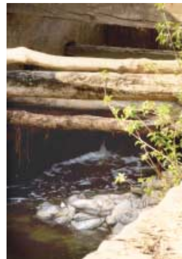
A sluice gate controlling a Khazans aquaculture system
