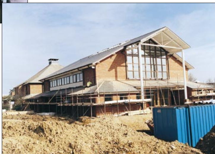
An extension to the Fowden Conference Hall, costing £1.2 million, was started in mid-August 1998 and is scheduled for completion in mid-Summer 1999. The new building will be named after Professor Trevor Lewis CBE, Director of IACR and of Rothamsted 1989-93. This major new facility will enable Rothamsted to host more international scientific conferences and will also provide an important local and regional venue for commercial seminars, training courses and trade exhibitions
