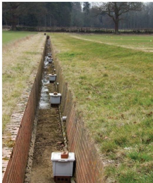
Drain outlets at eastern end of Broadbalk, 2010
