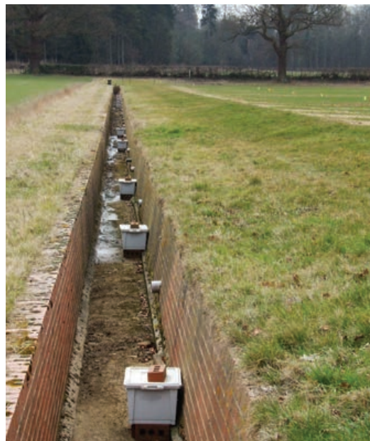
Drain outlets at eastern end of Broadbalk, 2010
