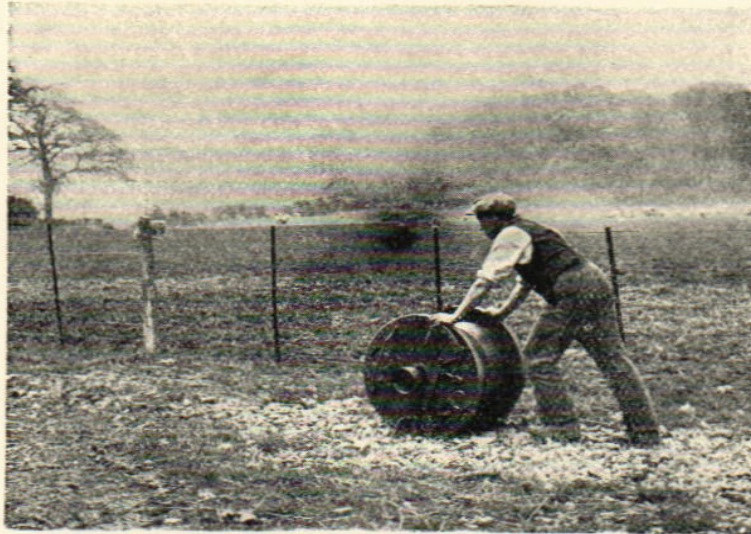
Fig. 10. 5 h.p. portable farm “ Drumotor ” in transit.
